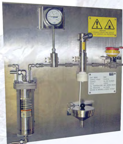
Panel mounted In-Line sample valve with In-Line heat exchanger to cool process media prior to it arriving at the sample valve, and temperature gauge.
